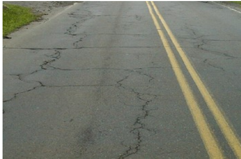
Cracking
