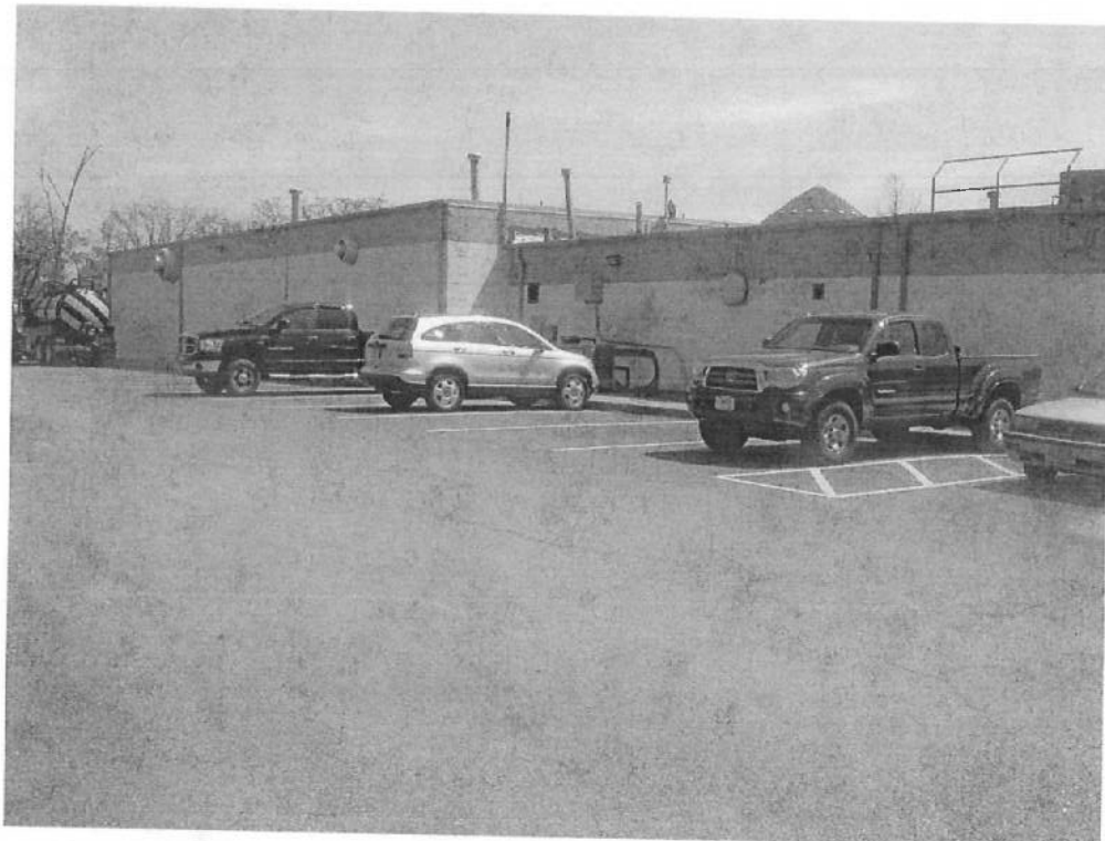
LBAM Building ID: 1324 Maintenance Office (Rear)
