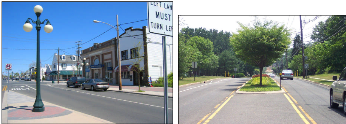
Main Street (Route 71) in Avon by the Sea (Monmouth County) and Federal City Road in Lawrence Township (Mercer County) provide good examples of “road diets.”
