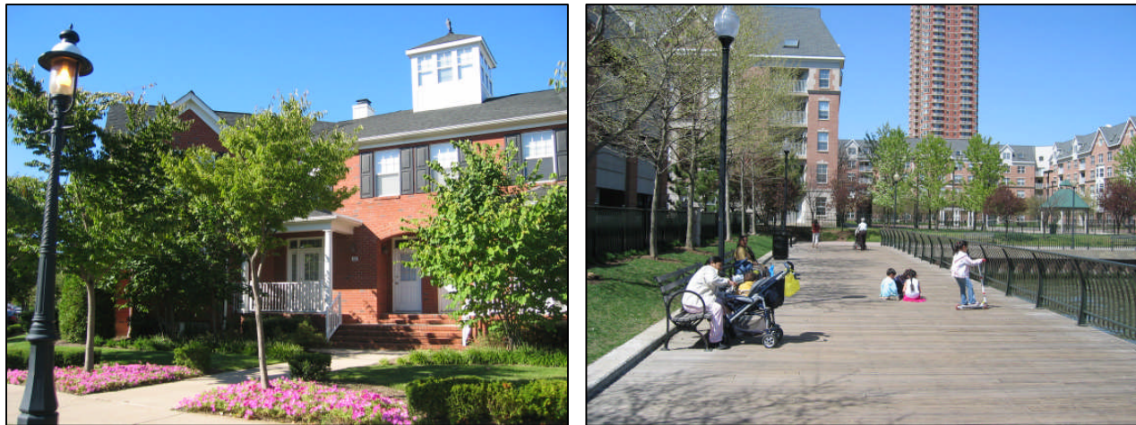
Attractive designs help generate community support for multi-family infill projects, like these in Metuchen (left) and Jersey City (right).
