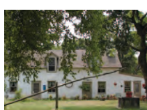
The John Holcombe House
