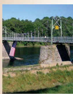
Lamberville-Raven Rock Pedestrian Bridge
