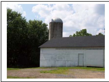
Silo and Barn, CR 524
