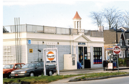
This gas station and convenience store in Massachusetts illustrates adaptive reuse with a free-standing sign that is compatible with the pedestrian environment in a town center.
