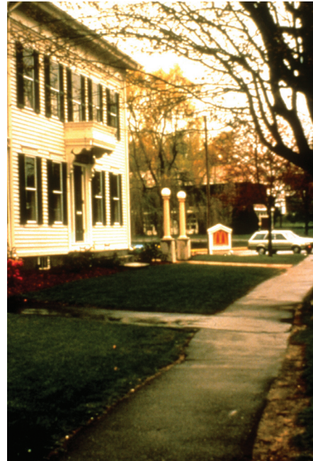
This McDonald's in Freeport, Maine is a good example of a adaptive reuse of a historic building and use of a monument sign.
