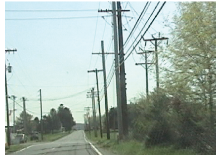
Utility clutter on Route 524 near Sharon Station Road.
