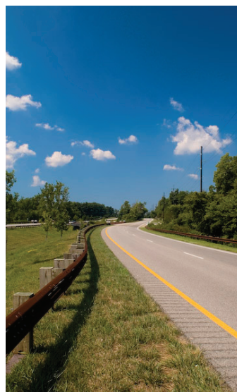
Example of a clear zone on Paris Pike in the Bluegrass Region outside Lexington, Kentucky. Notice how utility poles are set back away from the road (Source: americanbyways.com).
