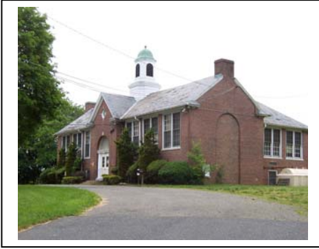
Imlaystown School, Davis Station Road
