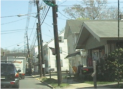
Utility clutter on Church Street in Allentown detracts from the Borough's historic character.
