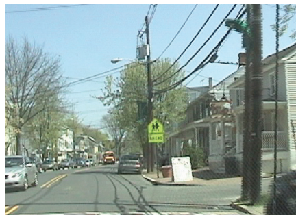
Utility clutter on Main Street in downtown Allentown.
