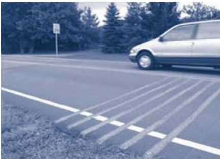
Bulb-outs at intersections with pedestrian activity (top photo) and rumble strips (bottom photo) along higher speed stretches of road that precede a known pedestrian area or crossing are possible traffic calming techniques for use along the Byway (Bottom photo source: http://www.dublin.oh.us/ ).
