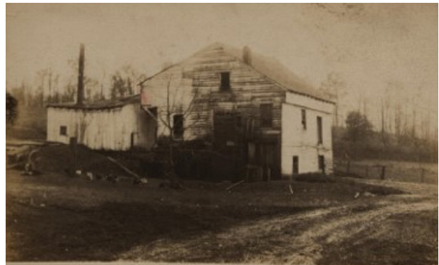
Historic site conditions
