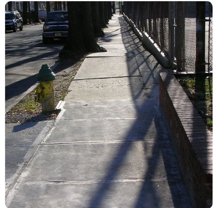
Good example: This well maintained sidewalk, which shows a recent repair, is safe for passage on foot or in a wheelchair. It sends the message that this space is highly cared for. Image: The RBA Group
