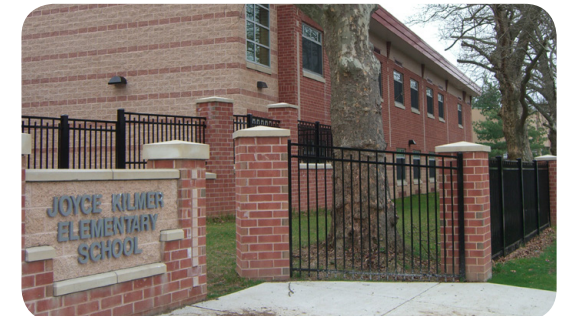
Good example: This painted aluminum fencing mounted on brick piers is both visually permeable and visually appealing. Its integration with the school's sign helps to underscore the importance of the school as an institution and a community. Image: The RBA Group
