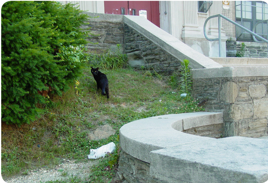
Poor example: This space adjacent to a school building shows signs of wear and offers little in the way of positive activity. Image: The RBA Group
