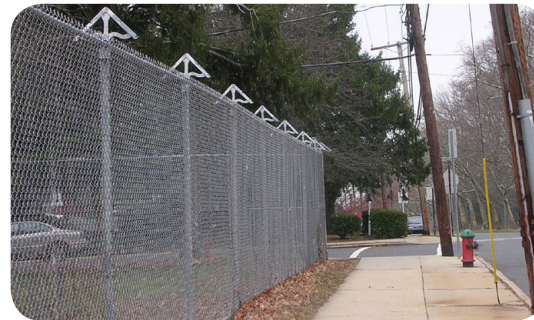
Poor example: Although this chain link fencing is visually permeable, the unfortunate side effect of its height, configuration, and barbed wire holders is an impression of the school as a prison-like facility. Image: The RBA Group
