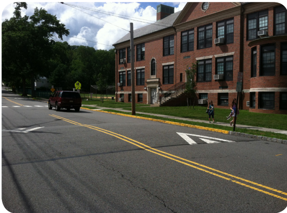
Speed hump in front of an elementary school in West Orange, NJ. Image: The RBA Group
