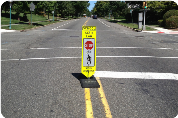
In-Street Stop for Pedestrians Sign with SCHOOL plaque mounted above the sign in Glen Ridge, NJ.
