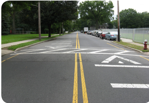
Raised crosswalk at Somerville School in Ridgewood, NJ. Image: The RBA Group
