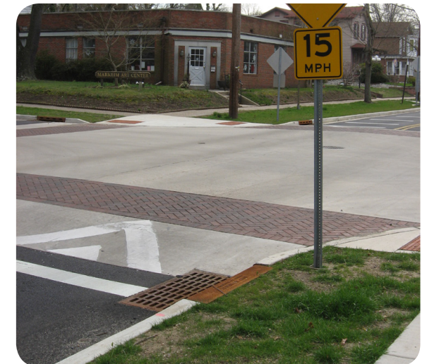
Raised intersection, Haddonfield, NJ. Image: VTC
