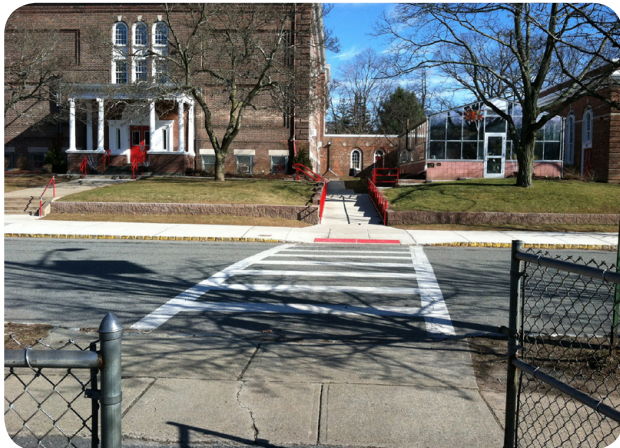
Fencing funnels pedestrians to the signed and well-marked mid-block crosswalk in front of the Watchung School in Montclair, NJ. Image: The RBA Group
