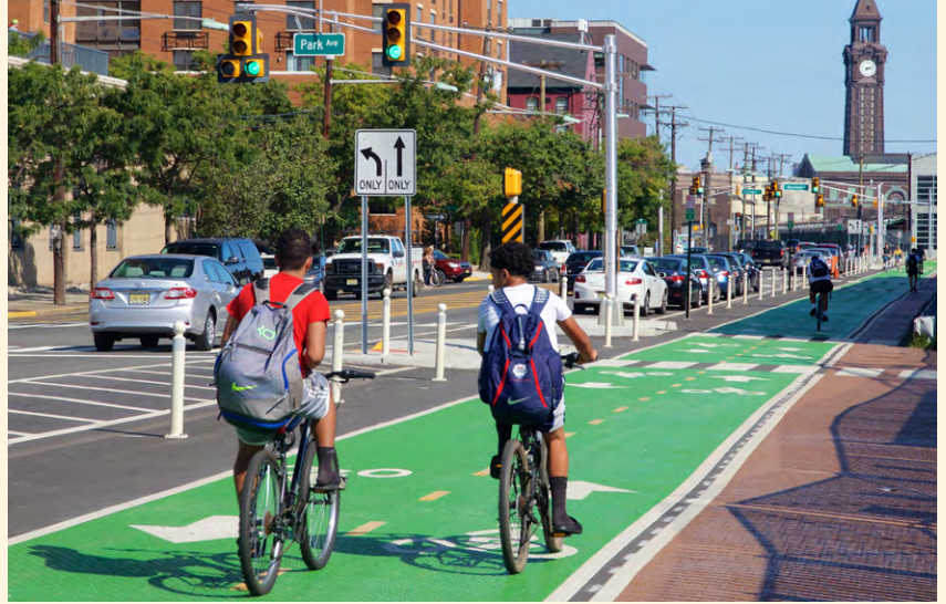
Two-way separated bicycle lane in Hoboken, NJ, with bollards and on-street parking separate bicyclists from motor vehicle travel lanes. Local preference can determine the use of a colored pavement treatment, as shown.
