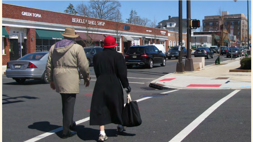
Signal heads with countdown timers clearly indicate when it is safe to cross the street and how much time pedestrians have to complete the crossing.
