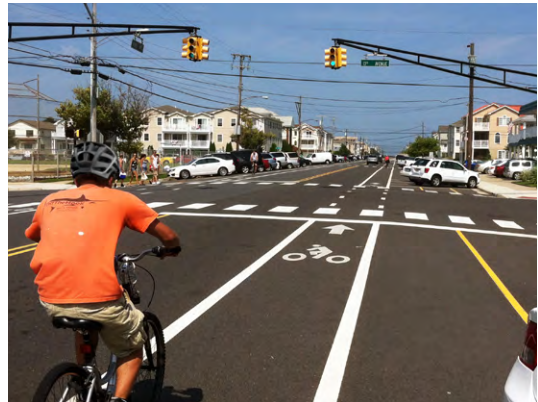
Bicycle lanes designate space for bicyclists through use of striping, pavement markings, and signs. They enable bicyclists to ride at their preferred speed without interference from motor vehicle traffic conditions and facilitate predictable behavior and movements among bicyclists and motorists.
