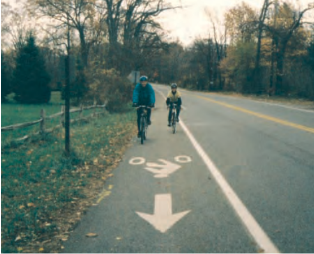
Bike Lane - A portion of the roadway designated by striping, signing and pavement markings that defines space for bicyclists
