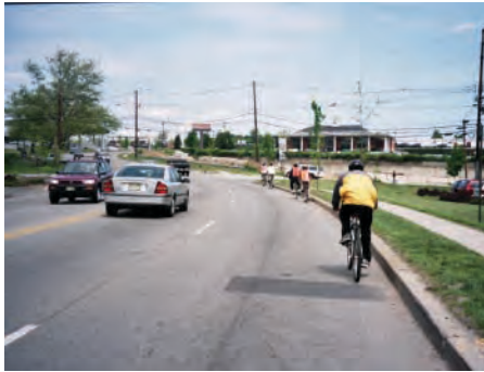
Shared Road - A roadway open to both bicycle and motor vehicle travel with wide curb lanes or paved shoulders
