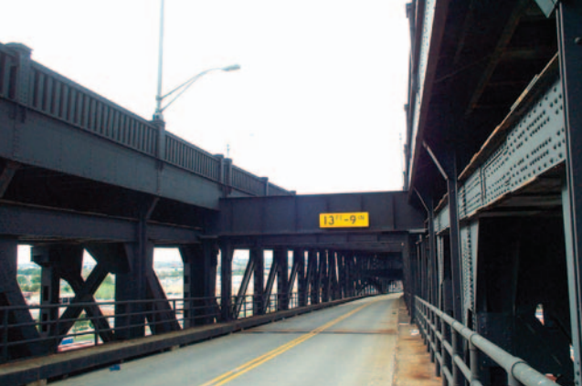
South Kearny Ramp, view looking west
