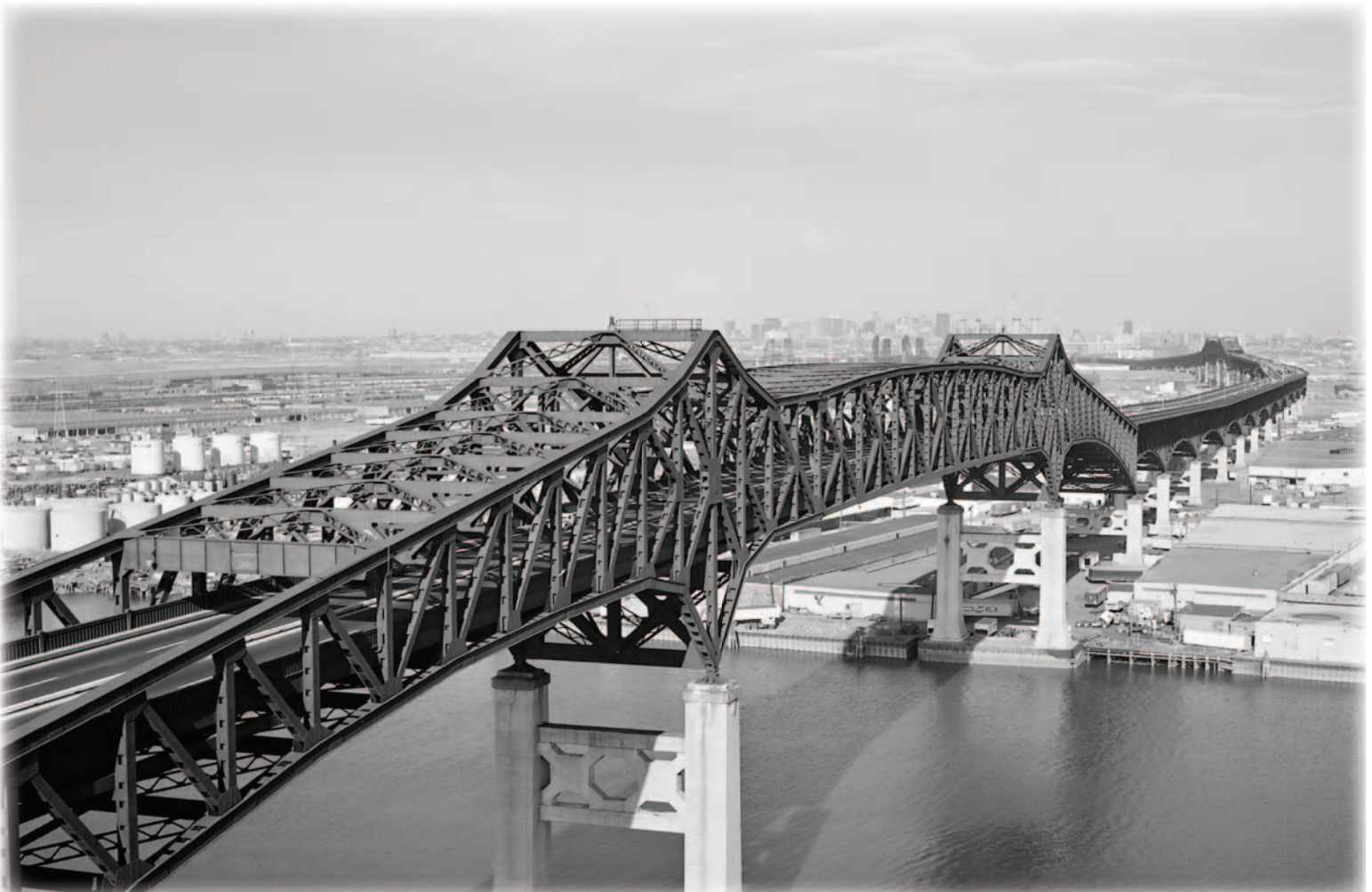
The Pulaski Skyway looking northeast over the Passaic River.
