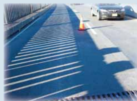
Completed deck overlay on eastbound roadway.
