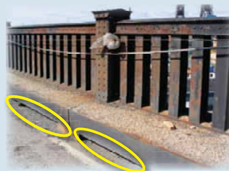
Repairs to the Skyway's drainage system are currently underway.
