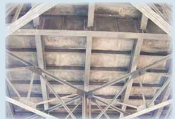
Underside view of the deck.
