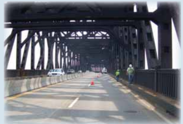
Eastbound deck and steel through truss.
