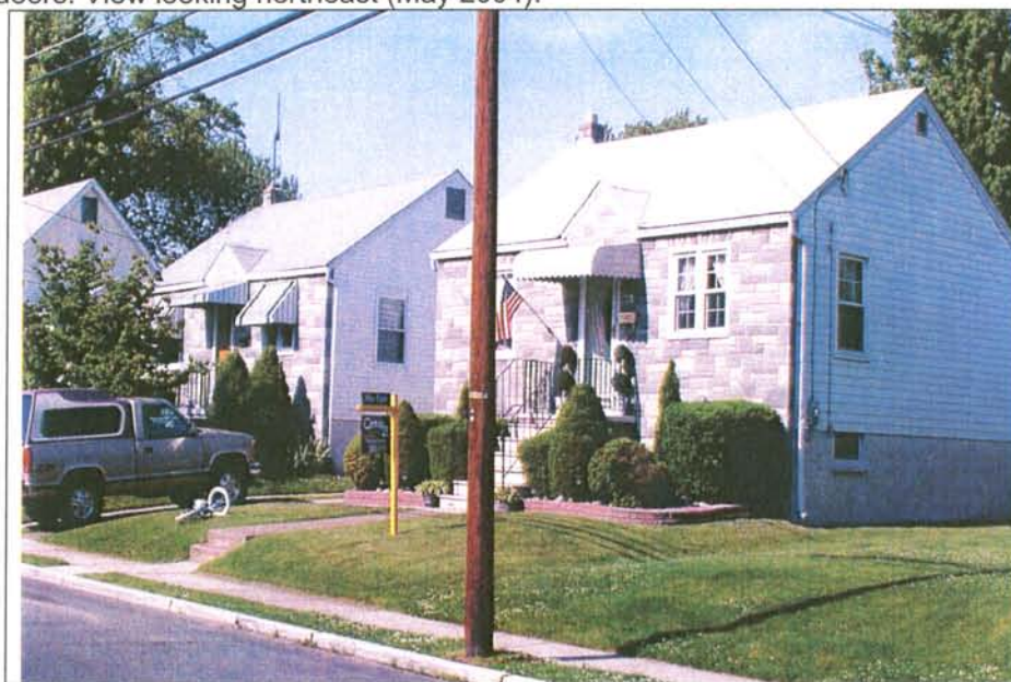
Photograph 1: 24-28 Harding Avenue. Note the gable wall dormers. Further note the replacement cladding, windows, and doors. View looking northeast (May 2004).
