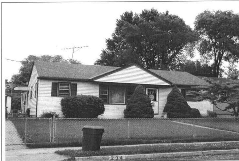
Photograph 1: 234 Lowell Avenue. Note the dual cladding and rear addition. View looking northwest (May 2004).
