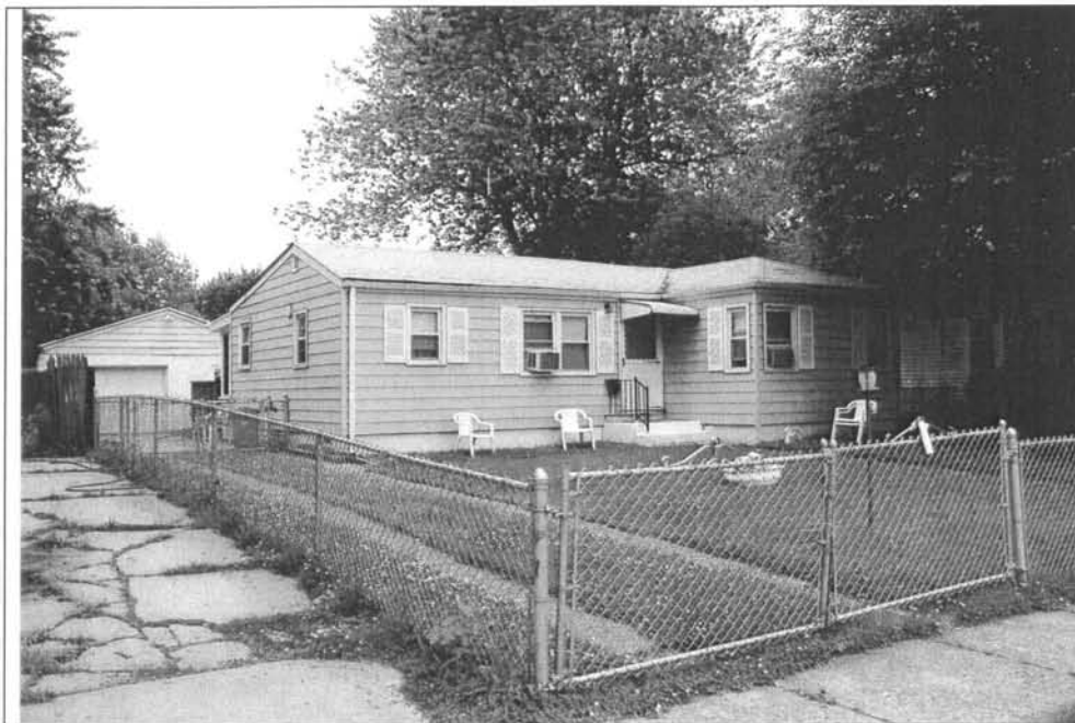
Photograph 2: 16 Cleveland Avenue. Note the modern rear addition. View looking east (May 2004).
