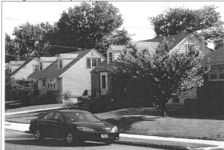
Photograph 1: 11-15 Baird Avenue. Note the gable dormers. Further note the modern cladding, windows, and doors. View looking southwest (May 2004).
