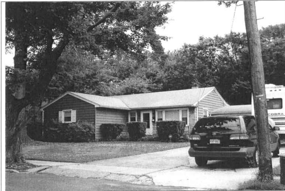
Photograph 2: 239 Lowell Avenue. Note the modern cladding, windows, and doors. View looking southeast (May 2004).
