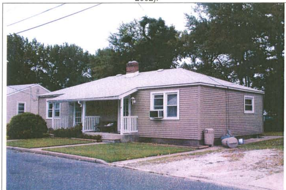
Photograph 1. Representative Type E dwelling with vinyl siding and replacement windows and doors (July 2002).
