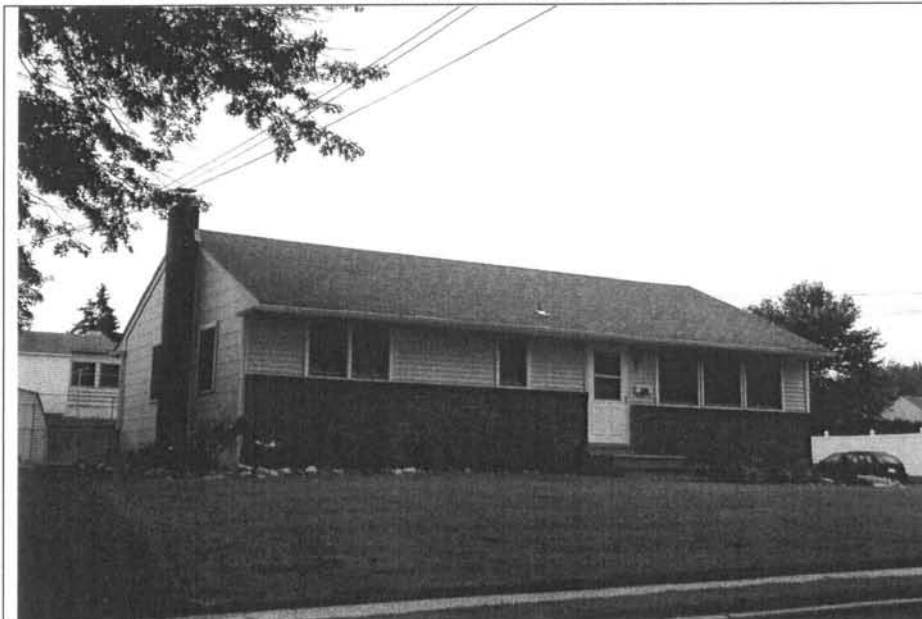
Photograph 1: 254 Lowell Avenue. Note the modern windows and doors. View looking north (May 2004).
