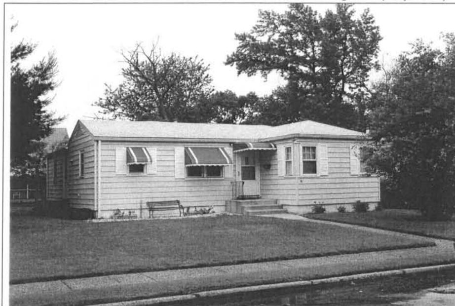
Photograph 1: 12 Roosevelt Avenue. Note the rear addition. View looking east (May 2004).
