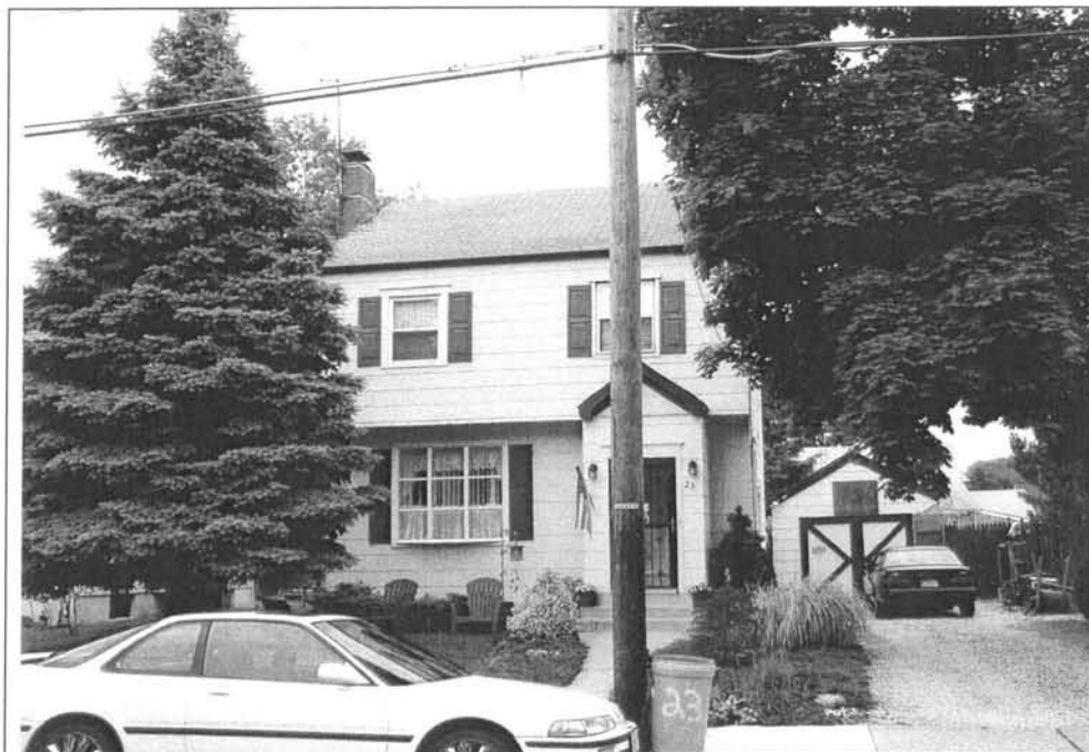
Photograph 3: 23 Adams Avenue. Note the enclosed entryway. View looking east (May 2004).
