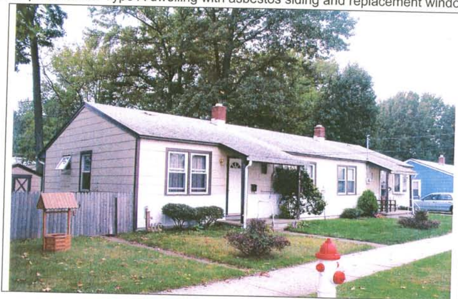
Photograph 1. Representative Type A dwelling with asbestos siding and replacement windows (July 2002).
