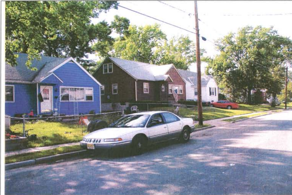
Photograph 2: Harding Avenue Streetscape. Note the replacement cladding, windows, and doors. View looking northwest (May 2004).
