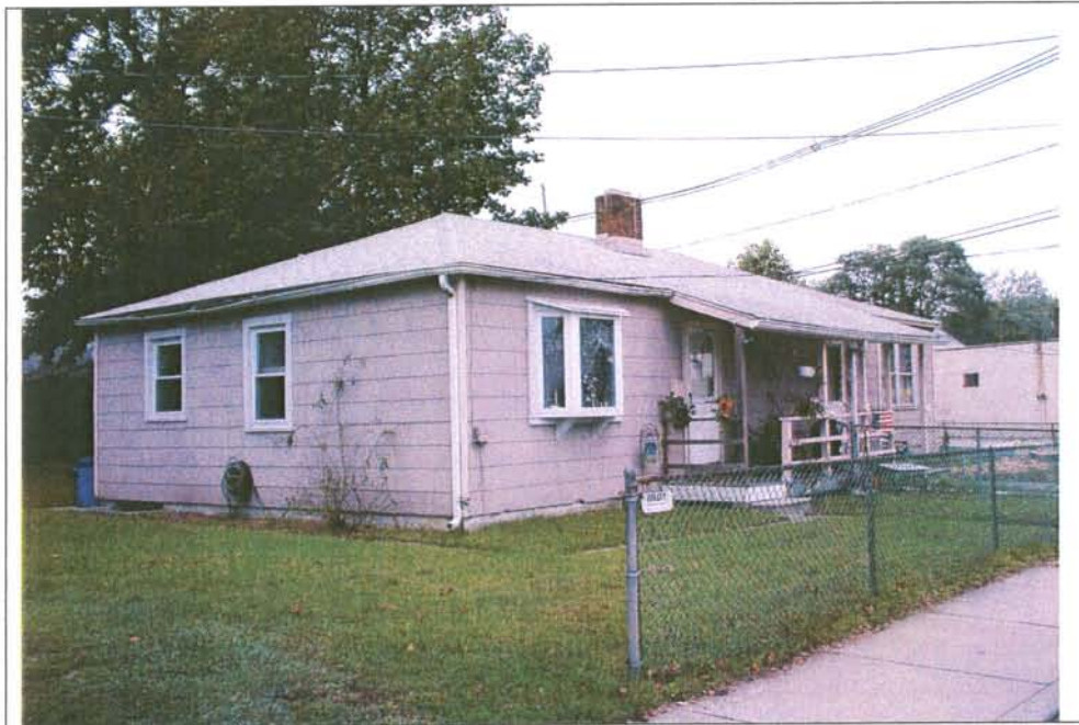
Photograph 3. Representative Type E dwelling with asbestos siding and modified windows (July 2002).
