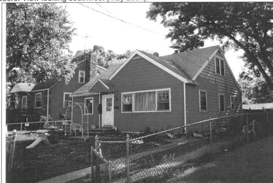
Photograph 1: 31 Harding Avenue. Note the large cross gable. Further note the replacement cladding, windows, and doors. View looking southwest (May 2004).
