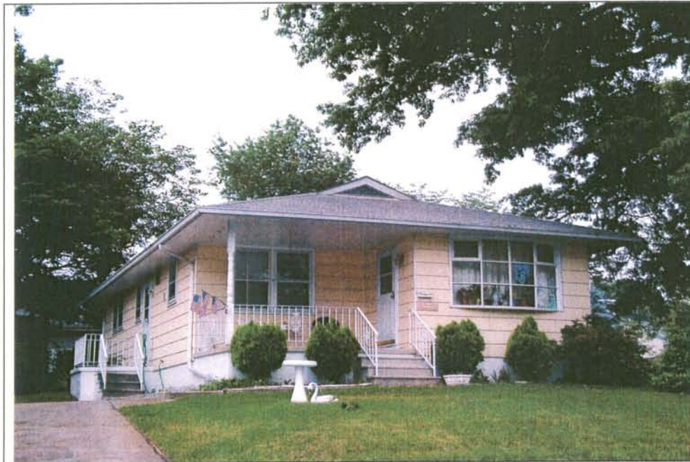
Photograph 2: 332 Lowell Avenue. Note the recessed entryway. View looking north (May 2004).
