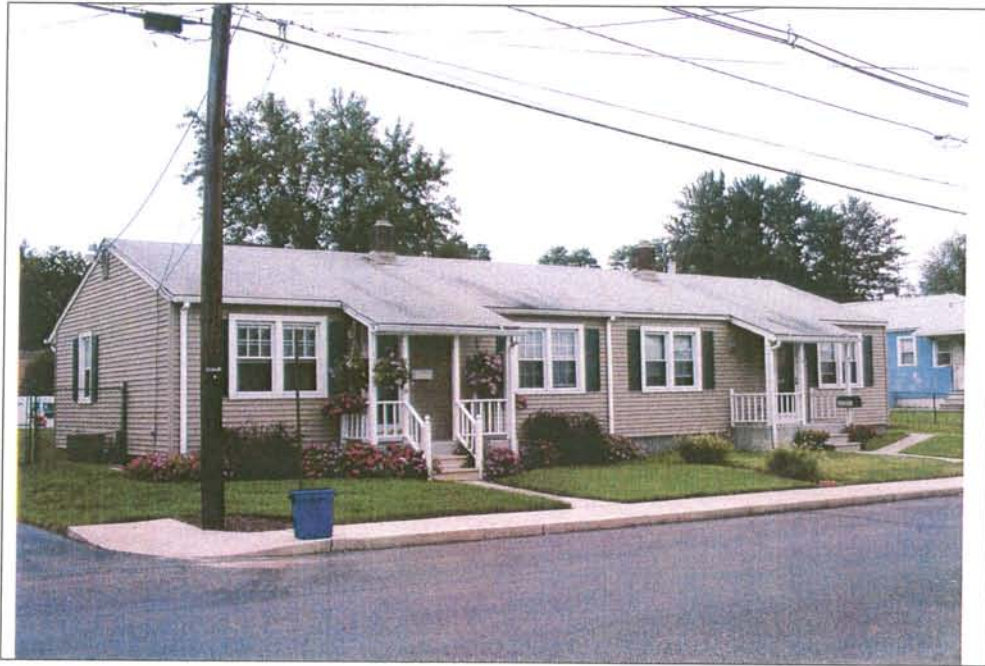
Photograph 2. Representative Type A dwelling with vinyl siding and replacement windows and doors (July 2002).
