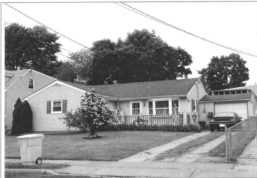
Photograph 3: 230 Lowell Avenue. Note the modern side addition, door, windows, and cladding. View looking northwest (May 2004).
