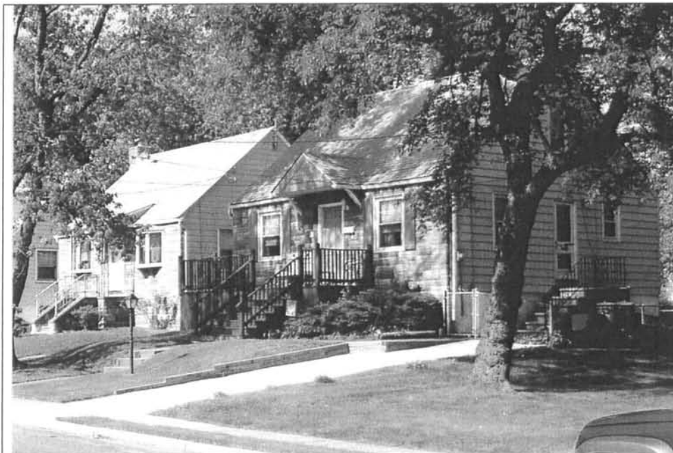
Photograph 2: Harding Avenue Streetscape. Note the original door and windows and the non-functional shutters. View looking north (May 2004).
