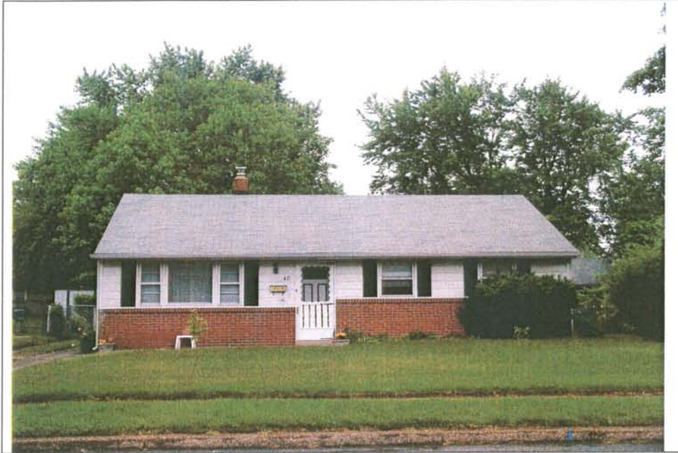
Photograph 2: 44 Midway Avenue. Note the original brick façade, windows and doors. View looking west (May 2004).
