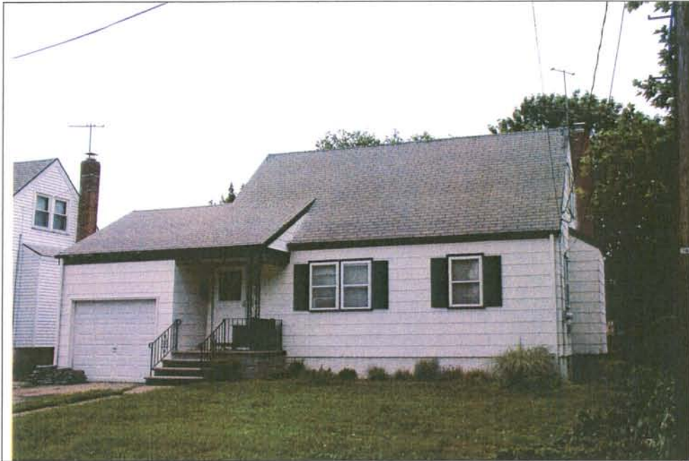
Photograph 2: 1137 Jefferson Avenue. Note the exterior brick chimney. View looking northeast (May 2004).
