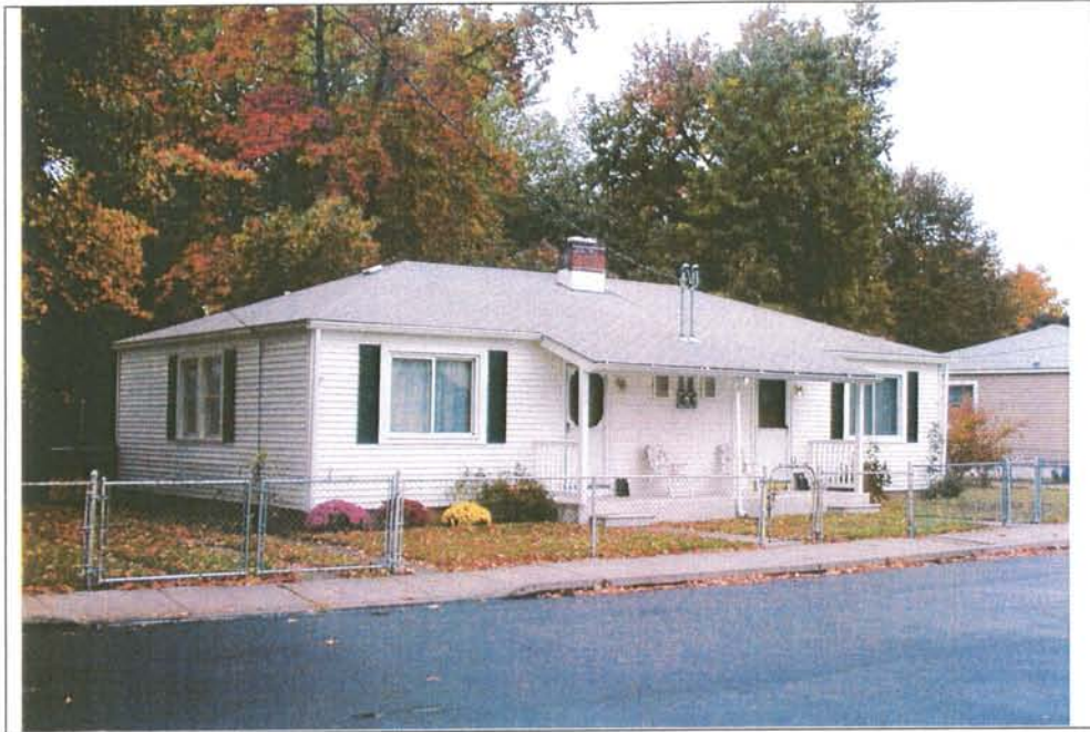
Photograph 2. Representative Type E dwelling with vinyl siding and modified windows (July 2002).
