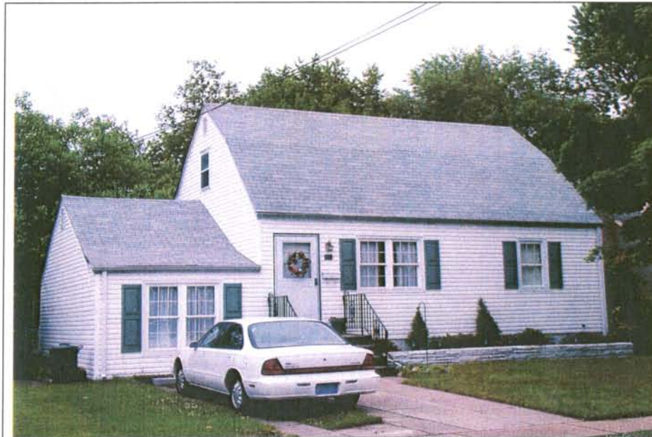
Photograph 1: 1156 Jefferson Avenue. Note the small side addition. View looking northwest (May 2004).
