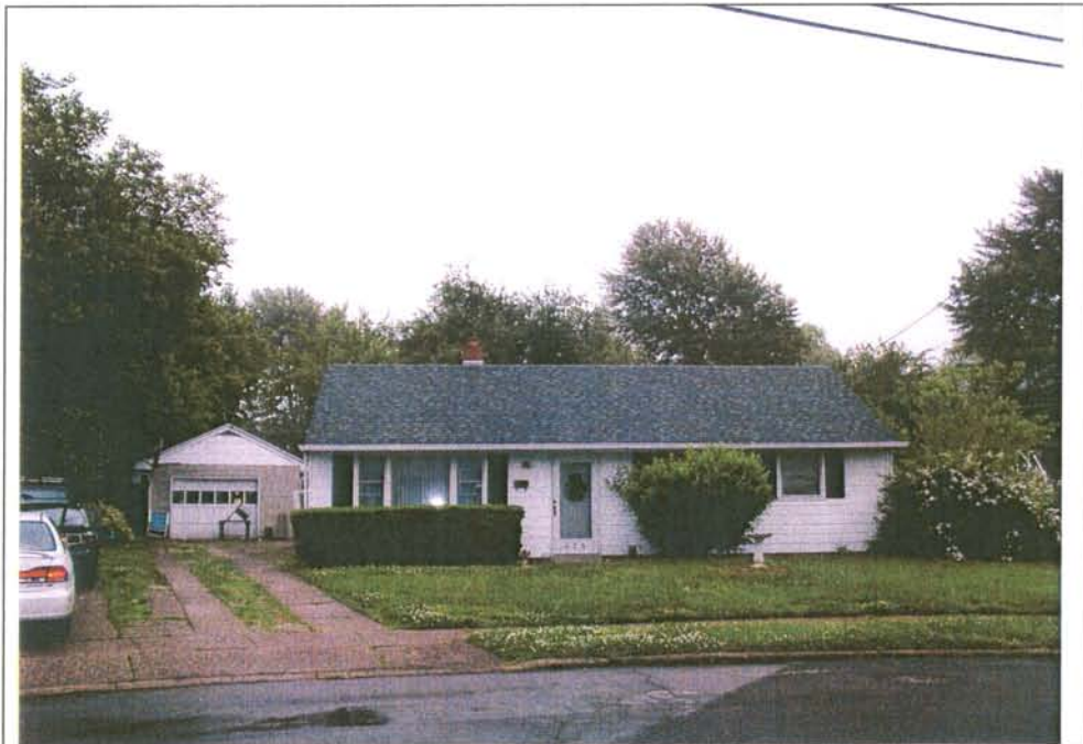
Photograph 3: 439 Dewey Road. Note the original cladding, doors, and windows. View looking northeast (May 2004).
