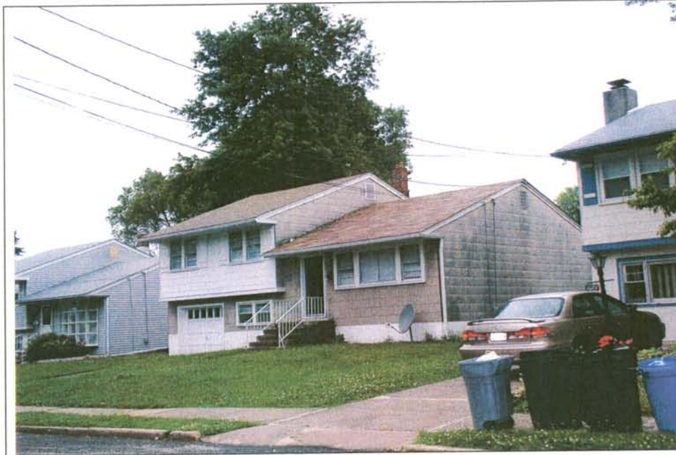
Photograph 2: 250 Lowell Avenue. Note the modern cladding and replacement windows. View looking west (May 2004).
