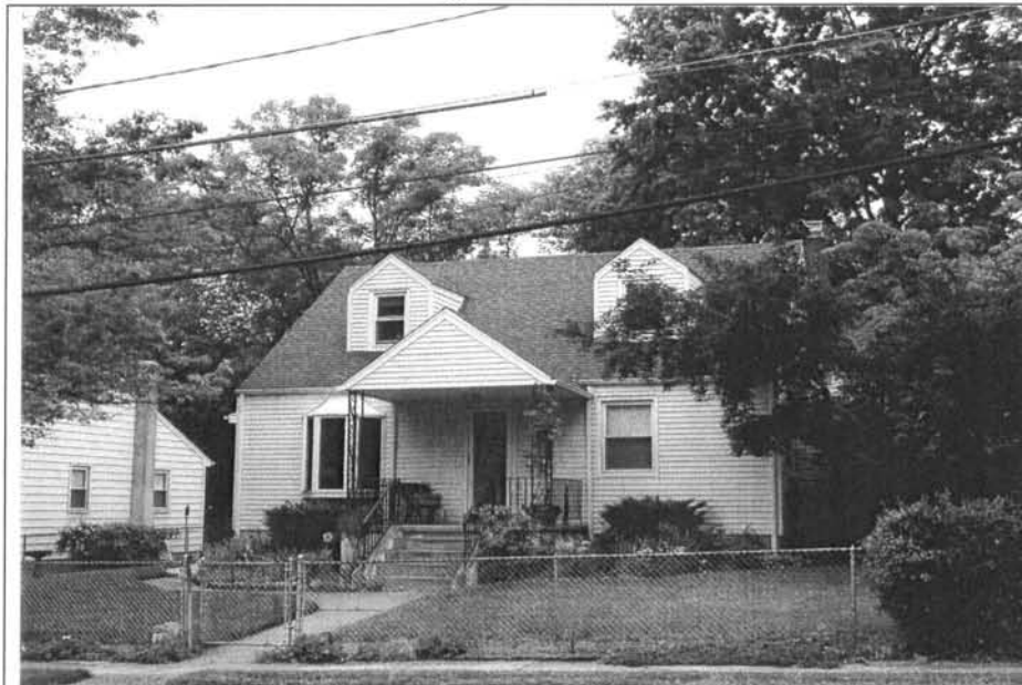
Photograph 1: 801 Bell Road. Note the modern gabled front porch. View looking southwest (May 2004).
