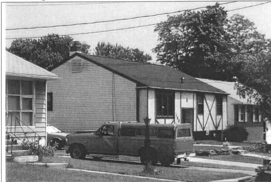
Photograph 1: 138 Harding Avenue. Note the modern façade. Facing northeast (May 2004).
