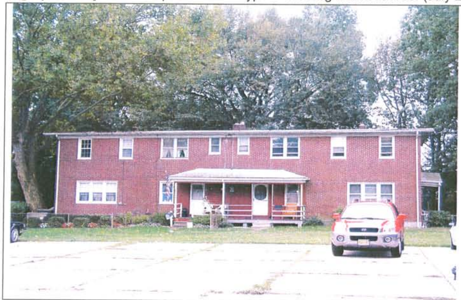
Photograph 1. Façade of a representative Type B dwelling with a flat roof (July 2002).
