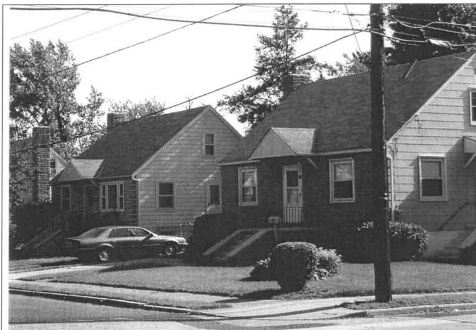
Photograph 3: Harding Avenue Streetscape. Note the modern cladding, doors, and windows. View looking southwest (May 2004).
