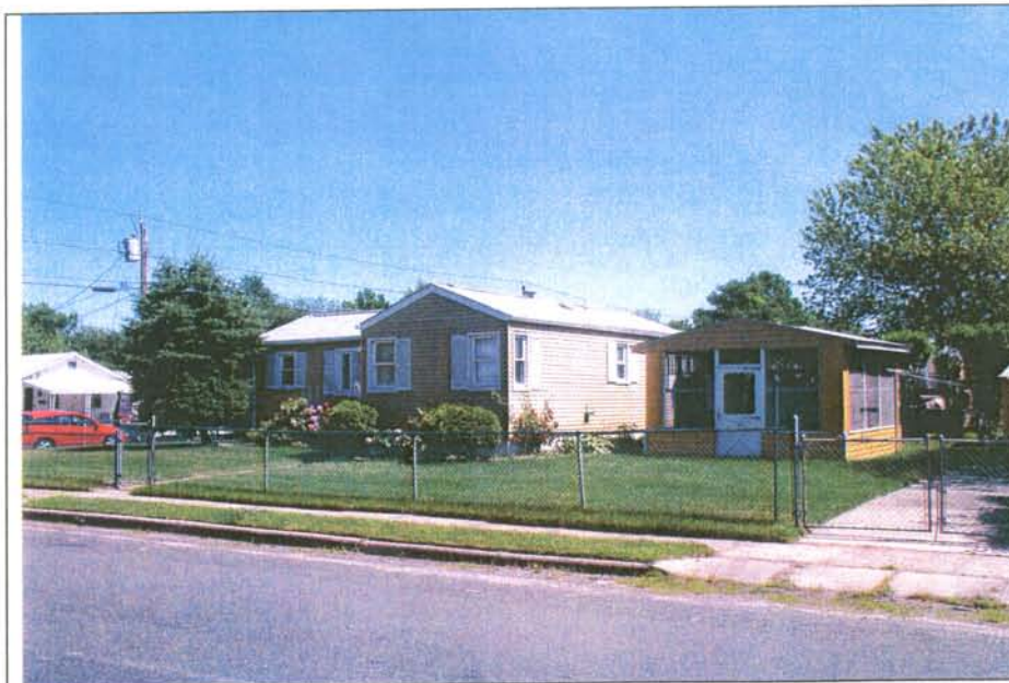
Photograph 1: 101 Linwood Avenue. Note the vinyl replacement windows and siding. View looking east (May 2004).
