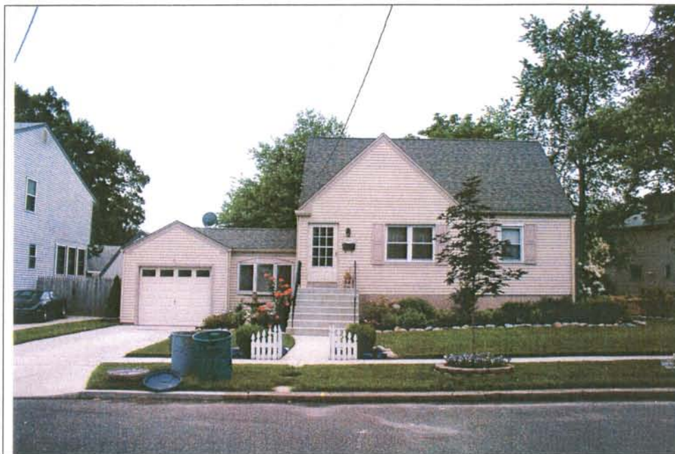
Photograph 2: 1018 Carter Avenue. Note the attached garage. View looking southwest (May 2004).
