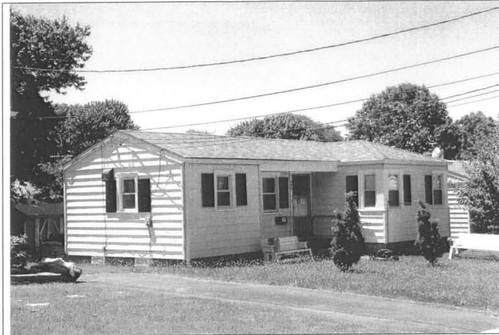
Photograph 2: 325 Baird Avenue. Note the replacement windows and doors. View looking west (May 2004).
