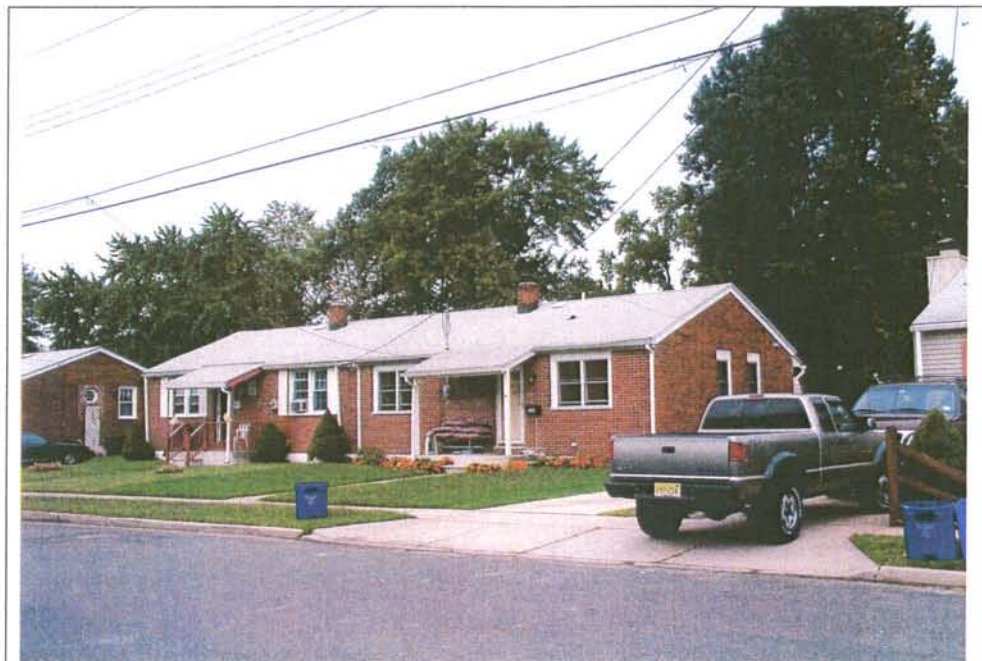
Photograph 2. Representative Type C dwelling with replacement windows and doors (July 2002).
