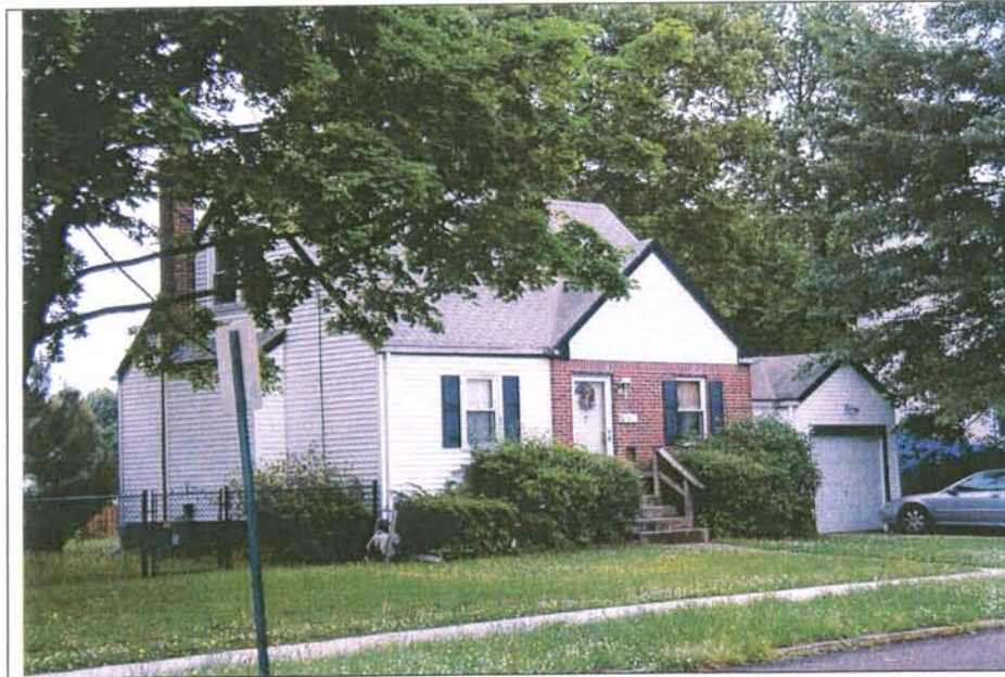
Photograph 1: 9 Park Drive. Note the modern replacement windows and door. View looking south (May 2004).
