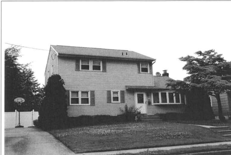
Photograph 2: 304 Lowell Avenue. Note the modern, second-story addition, cladding, windows, and doors. View looking north (May 2004).
