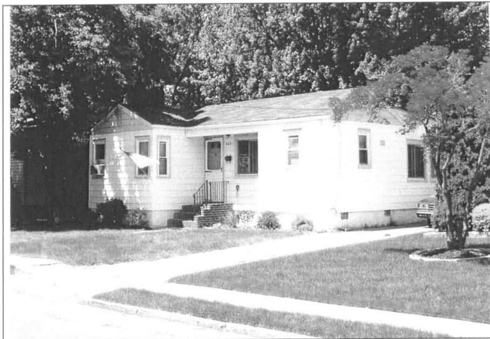
Photograph 3: 206 Lincoln Avenue. Note the modern door, windows, and cladding. View looking east (May 2004).
