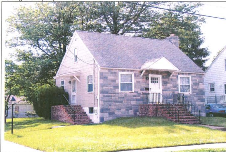
Photograph 1: 55 Harding Avenue. Note the Permastone cladding. Further note the original doors and windows. View looking north (May 2004).
