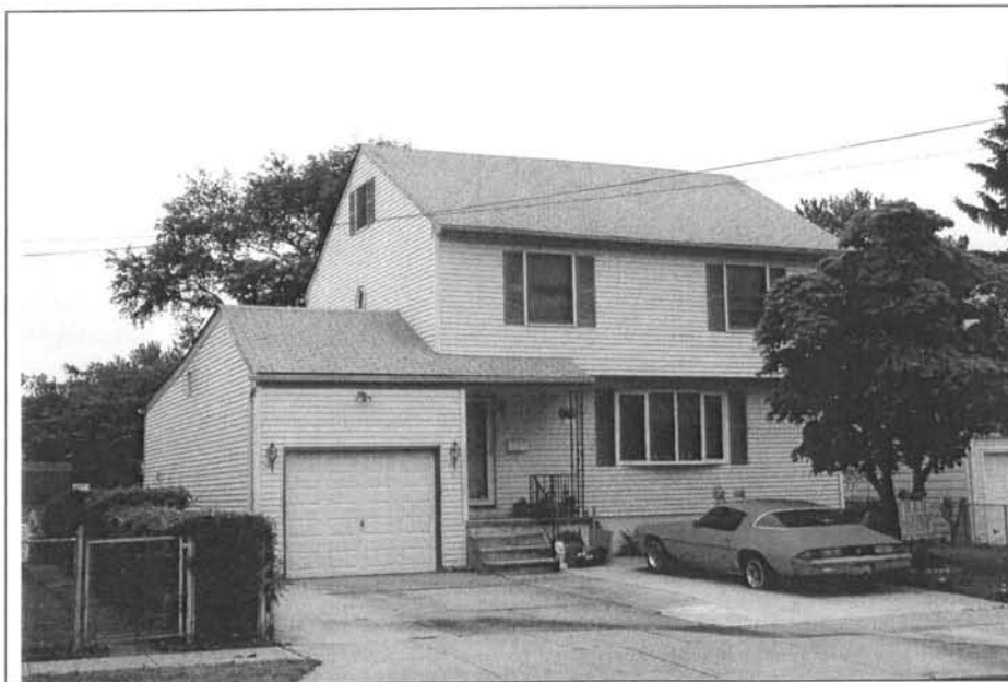
Photograph 1: 3 Bergen Avenue. Note the attached garage and recessed porch. View looking southeast (May 2004).
