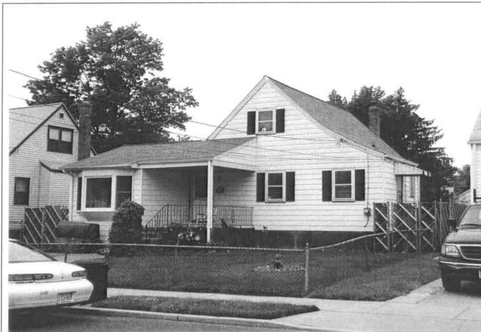
Photograph 3: 18 Monroe Avenue. Note the shed roof porch. View looking north (May 2004).
