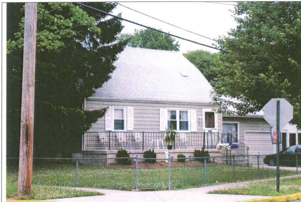
Photograph 2: 14 Bergen Avenue. Note the original pane-and-panel door and the modern side addition. View looking north (May 2004).
