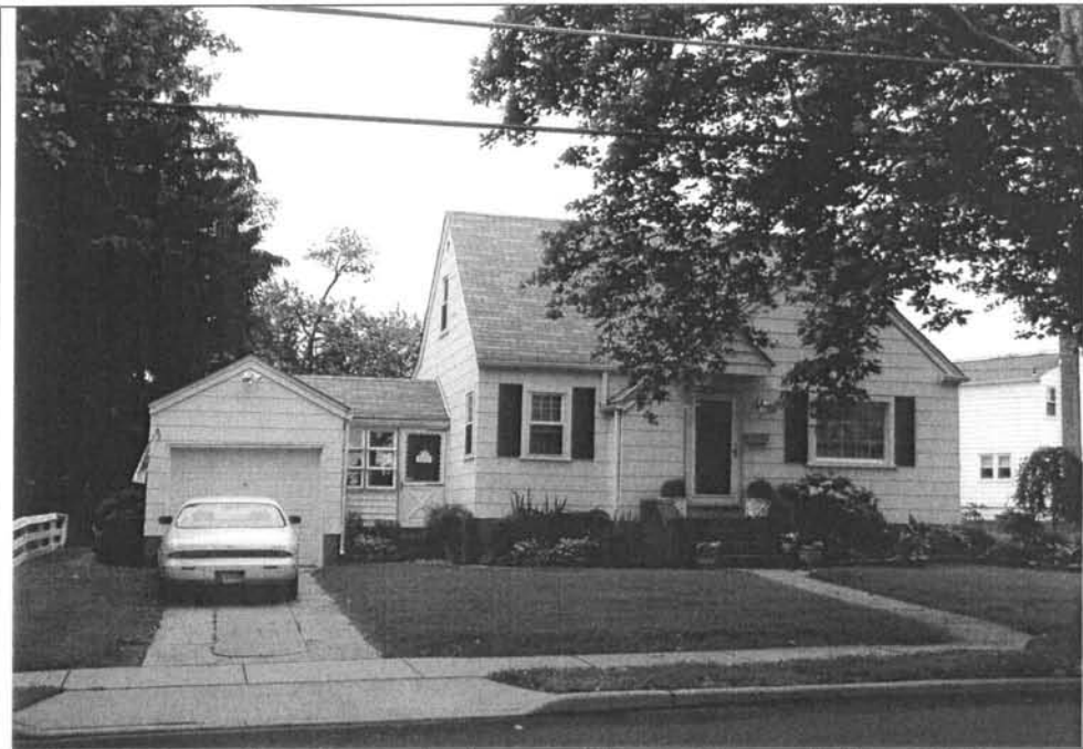
Photograph 3: 6 Union Avenue. Note the attached garage. View looking north (May 2004).
