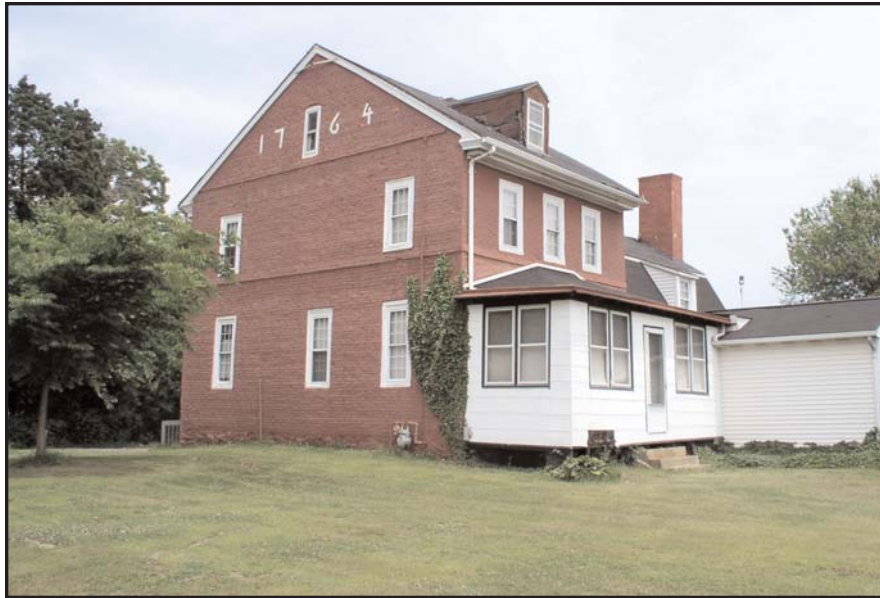
Plate 3: Harrison-Glover House. View looking northeast (June 2004).
