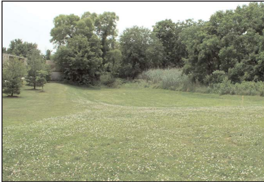
Plate 1: Stormwater retention basin in Area I. View looking south (June 2004).
