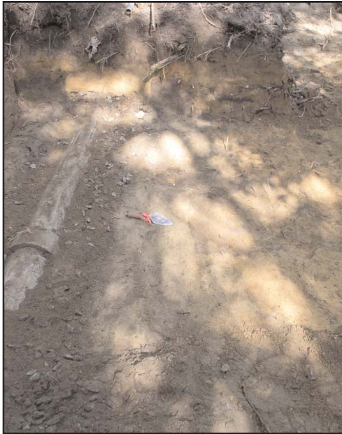
Plate 7: Fiberglass coated pipeline in Trench 1A. View looking northwest (May 2005).
