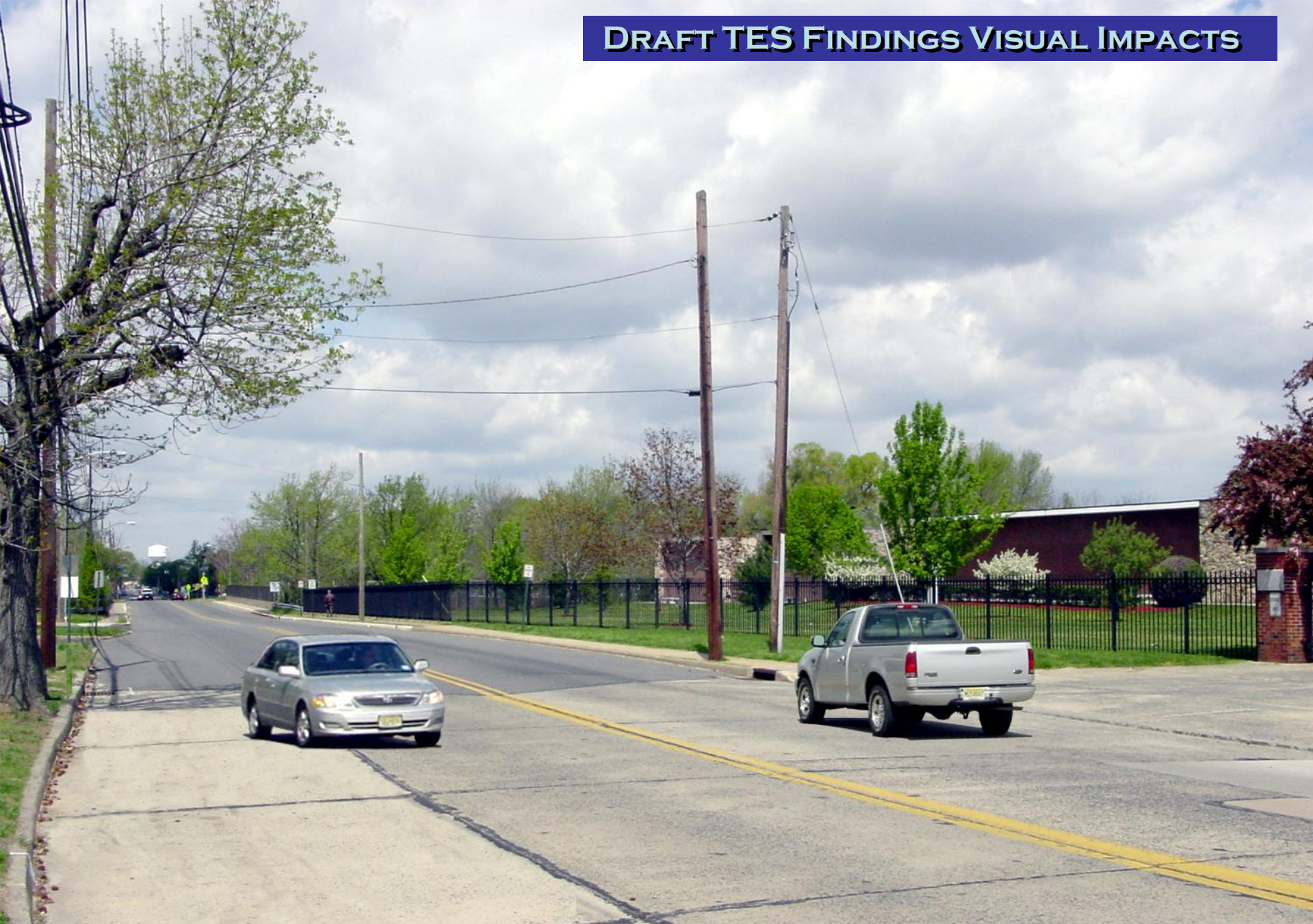
BROWNING ROAD LOOKING WEST - EXISTING CONDITIONS
