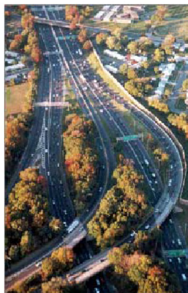
Aerial view of the I-295/I-76/Route 42 Interchange.
