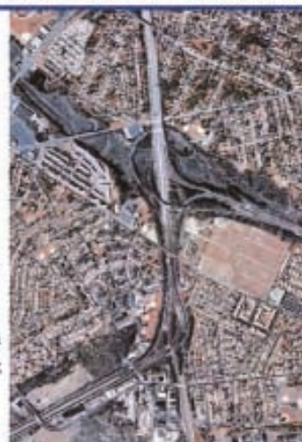
Source: NJDEP Bureau of Geographic Information and Analysis, Current aerial of I-295/I-76/Route 42 Interchange
