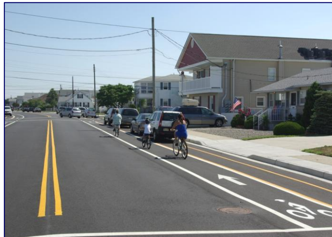
This striped bicycle lane fits the local context, improves safety and mobility, and Completes the Street in Wildwood, NJ
