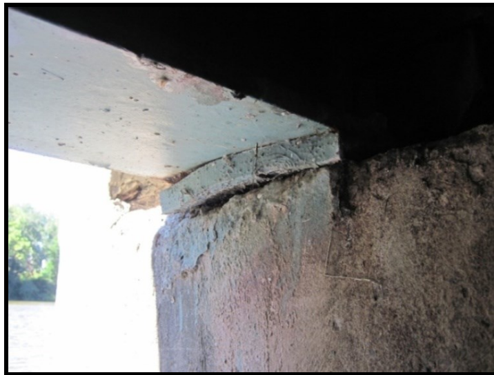
Figure B.1.4—South Fascia Elastomeric Bearing
