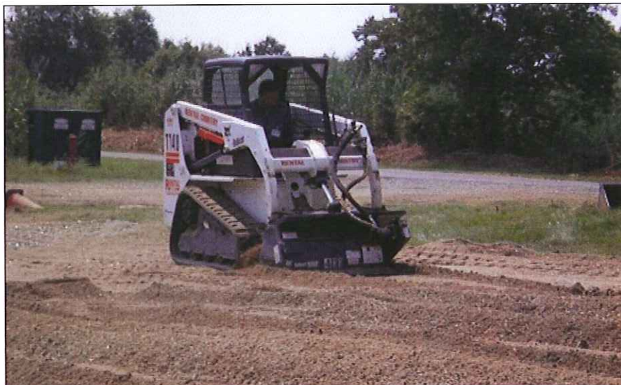
Figure 12. Bobcat used to mix separated sandy material with recycled glass.
