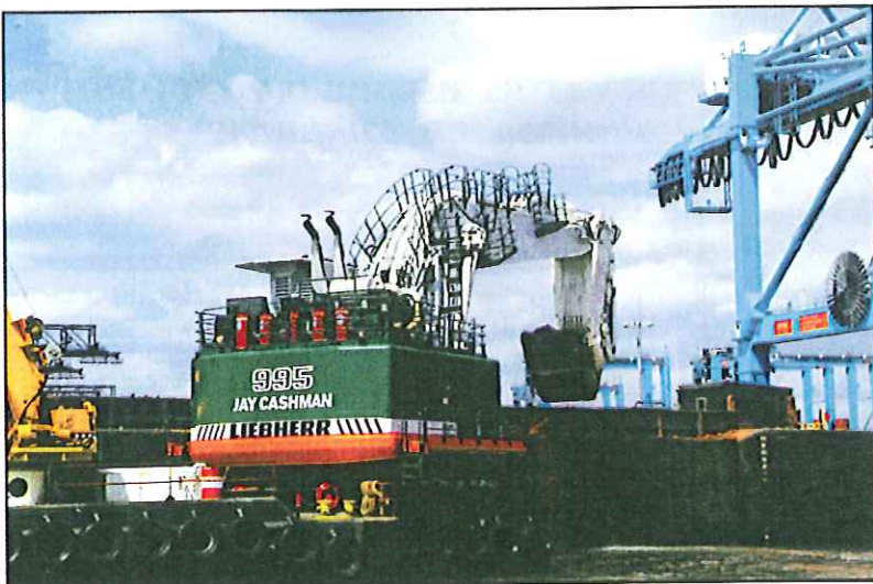
The backhoe dredge Jay Cashman digging in Newark Bay, April 2004.
