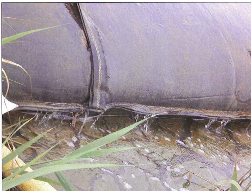
Figure 16. Decant water draining from geotextile tube.
