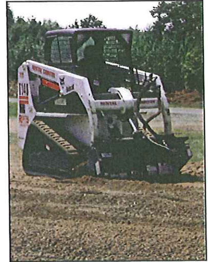
Mixing the sand and glass with a rotary tiller. Photo by Edward Gorleski, OCC
