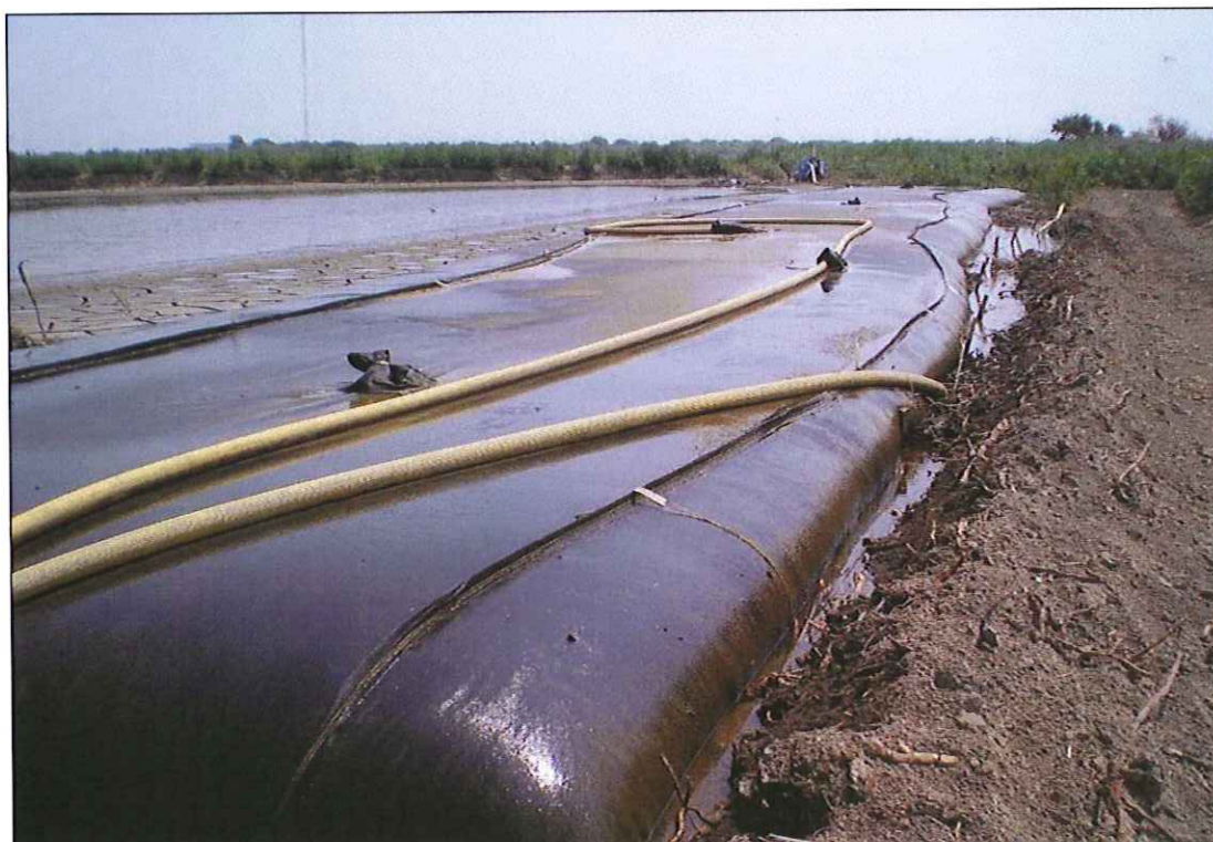
Figure 14. Dewatering Geotextile Tube
