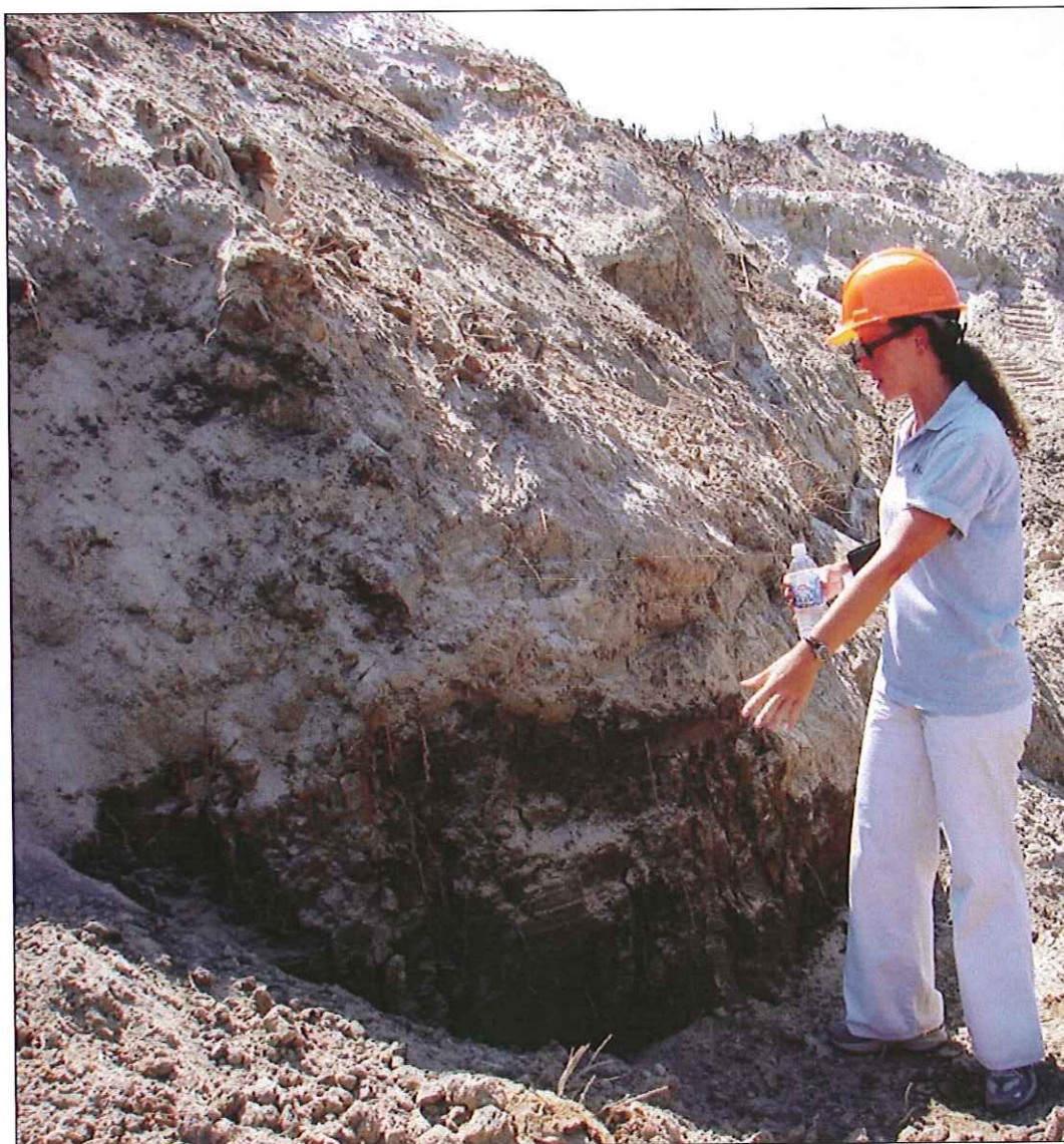
Figure 3. Layers of sand and silt/clay material can be observed in Site #3 after excavation.
