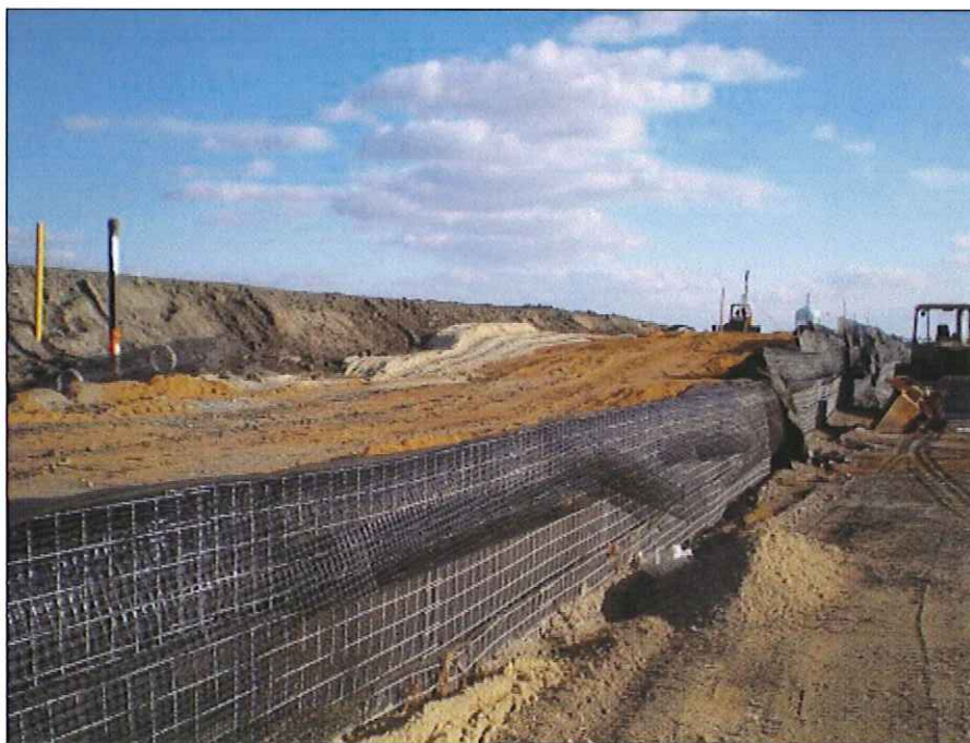
Figure 19. Ramp construction at the Route 52 causeway reconstruction project.
