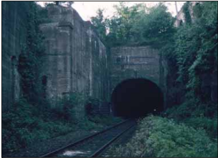
East Portal of the Bergen Tunnel
