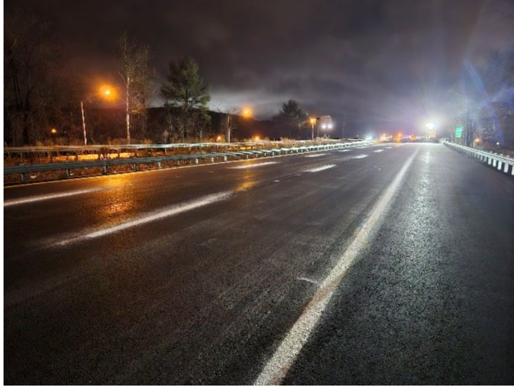
Newly paved roadway
