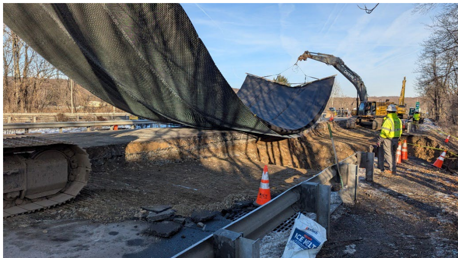
Installing wire mesh
