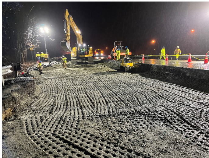
Backfill and compaction
