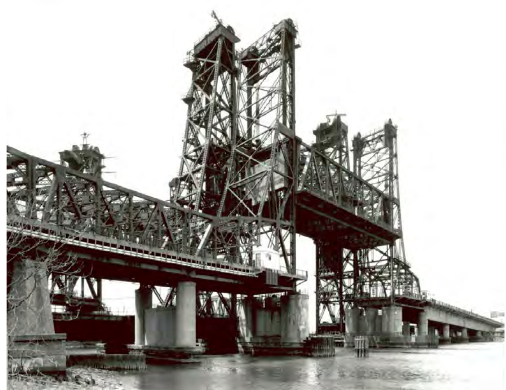
The Wittpenn Bridge in 2005 in the open position (Elliott 2005).
