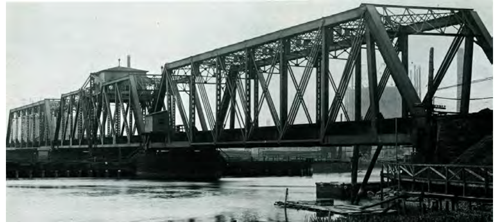
Undated photograph of the Delaware, Lackawanna & Western Railroad's swing span bridge over the Hackensack River, built in 1902 (Taber).
