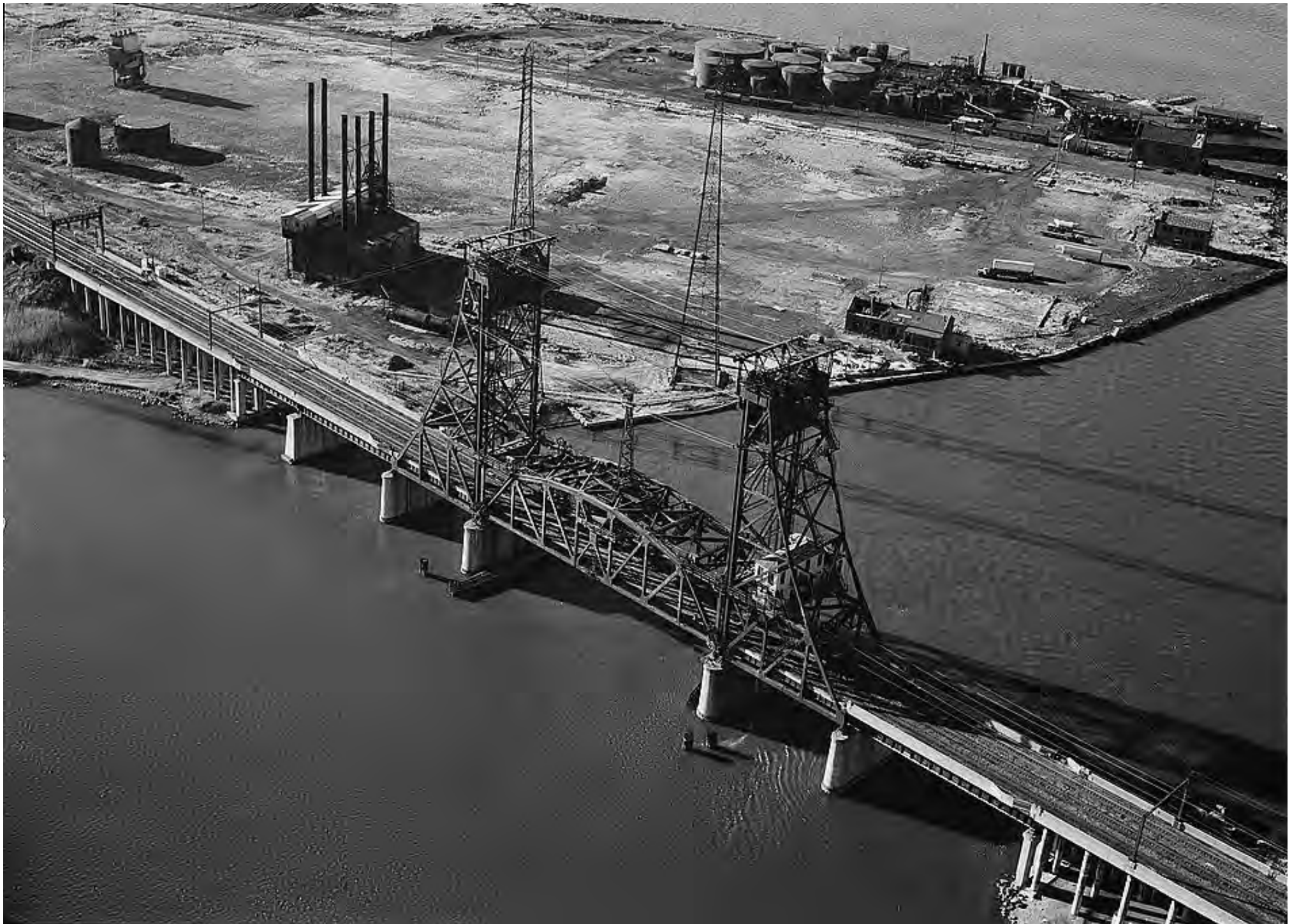
The DL&W's Hackensack River Bridge, known as the Lower Hack, in 1979 (Boucher, HAER-Erie & Lackawanna Railroad Bridge).
