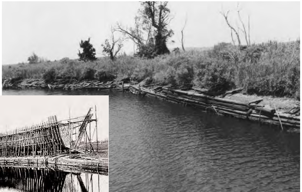
Looking downstream on Dennis Creek at low tide from the Route 47 bridge toward the site of the Diverty shipyard; two others were nearby. Remains of wooden bulkheads and cribbing are visible along the north bank at right. Inset: A schooner takes shape at the shipyard in this historic photograph [Sources: Hunter Research, Inc.; George Brewer, Jr.].
